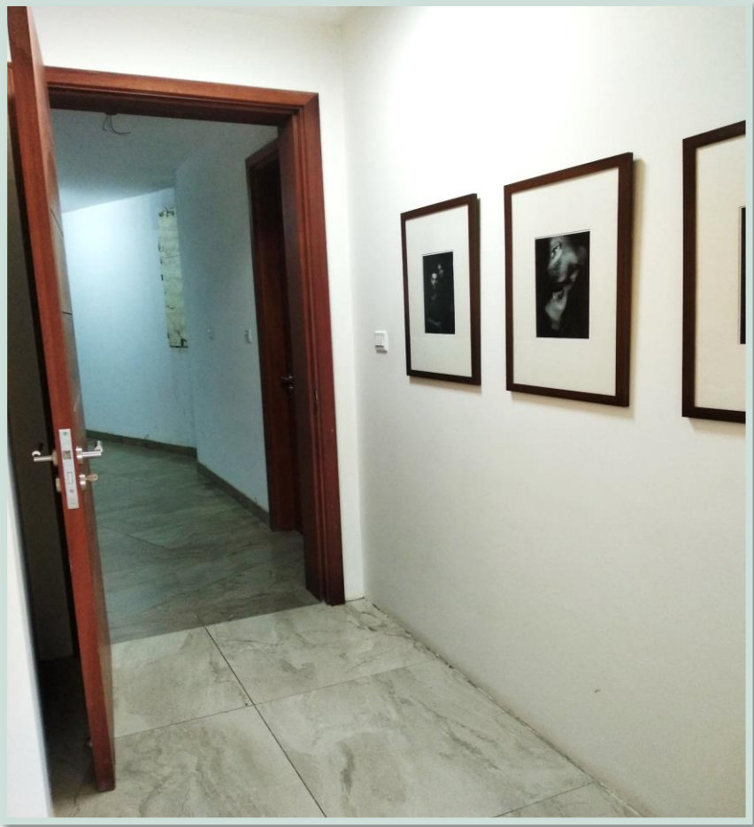
Fig 18. Hallway Tilework - 1st Grade full bodied porcelain & rectified Spanish made tiles
